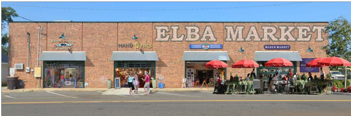
Elba, AL (Proposed Conditions): The building is quite wide, therefore, it is recommended that four bays be punched through the side facade and demising walls be constructed on the interior to create four micro-retail venues. Consider using roll-up garage doors with glass inserts that can be rolled up during nice weather. When too hot or cold, keep them rolled down but include a regular door to the side to access each retail space. Metal canopies, signage and gooseneck lights all work together to break up the long, blank facade. Consider painting an intentionally distressed sign like “Elba Market” as shown above to create a sense of age to the building.
